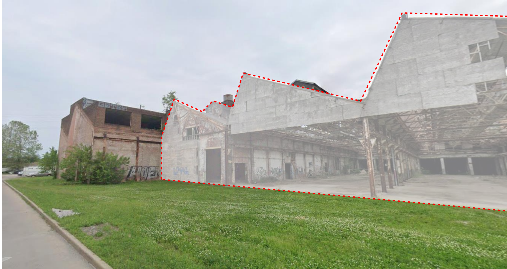
Existing Building 6 & Sheds (To be Demolished)
