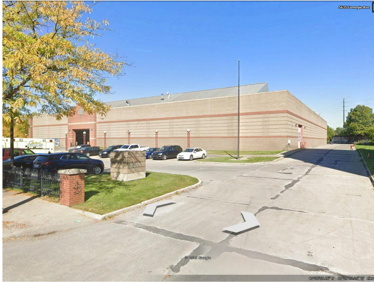
Equipment Service Station - West
