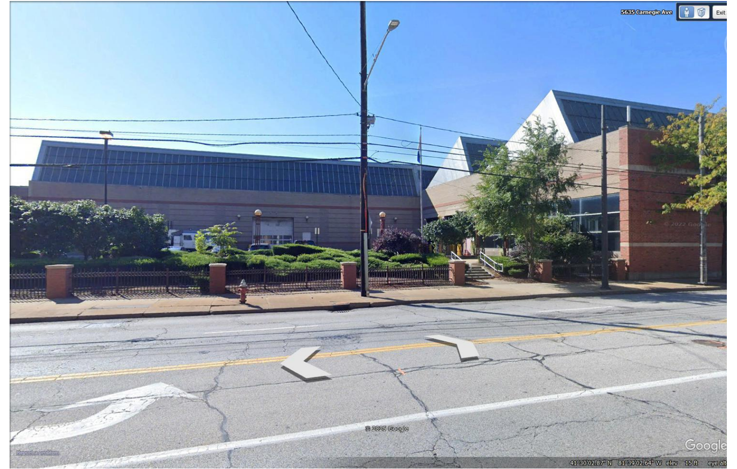
City of Cleveland Building – Waste Management - Southwest
